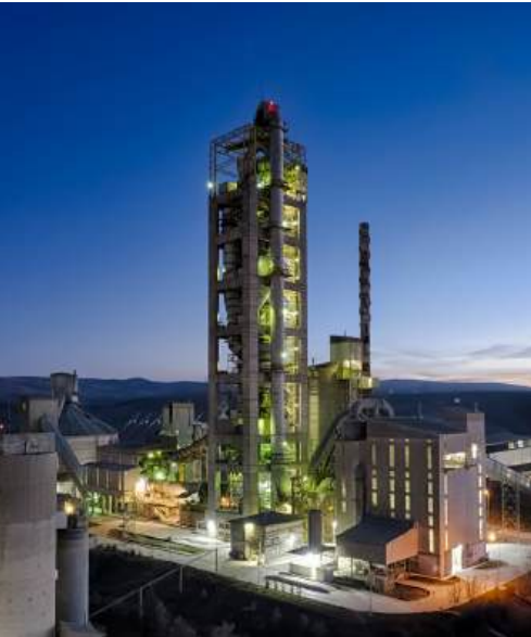
Votorantim Cimentos has pioneered in Turkey the use of biomass waste. At its Yozgat plant the alternative fuel in the main burner is primarily corn stalks. At its Hasanoğlu plant, biomass is used in the calciner line. Read more on p83
