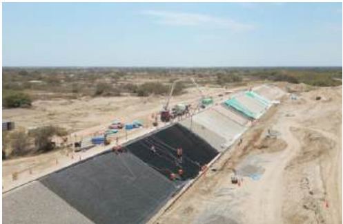
Cementos Pacasmayo in Peru has extended Cement Soil Stabilisation beyond pavements into riverbank defences to protect vulnerable communities from extreme weather events, saving 20% of CO 2 emissions. Read more on p46
